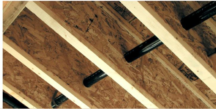
I-JOIST 301 MM LUZ MAXIMA 5.50 MTS @ 40 CMS PARA CARGAS DE 250 KGS/M2
