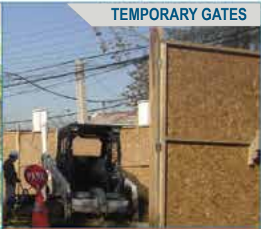
JOB SITE STRUCTURES
